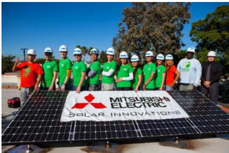
Mitsubishi Electric volunteers and University students installed the solar system.
